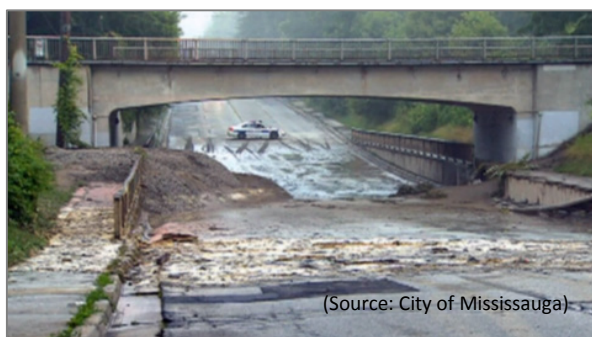
Figure 6: ROW impact of July 8, 2013 storm in Mississauga
