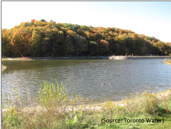
Figure 4: Earl Bales Park Stormwater Pond
