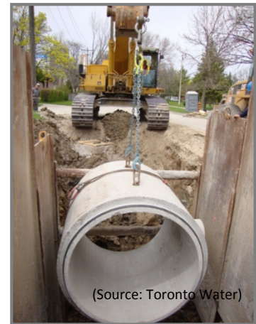
Figure 3: Storm sewer upgrades for areas with basement flooding
