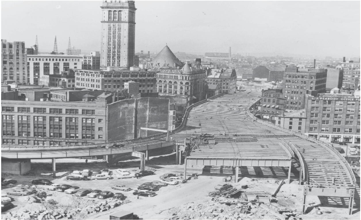
Figure 19 Construction of Boston Central Artery circa 1956 (Brown, Morris and Taylor, 2009)
