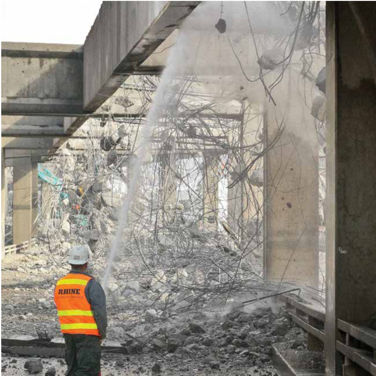
Figure 10 Teardown of the Alaskan Way Viaduct, Seattle (Washington DOT, 2014)
