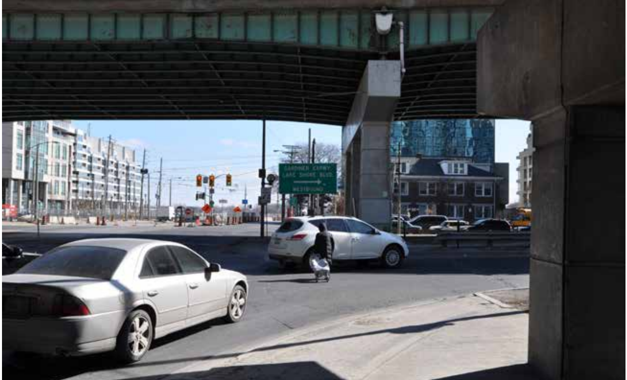
Figure 32 Lack of accomodation for pedestrians results in unsafe crossing. (Gordon, 2014)
