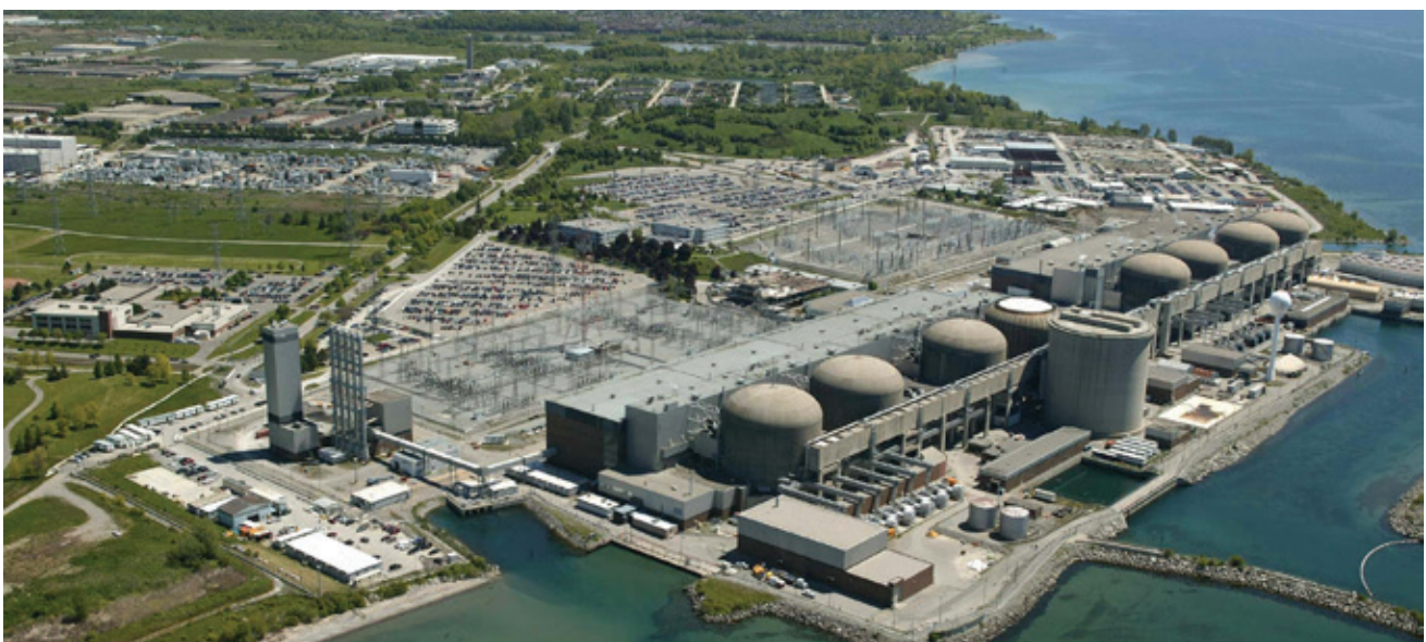
FIGURE 1: An aerial image of the Pickering Nuclear Generating Station, 2010 (Image source: Ontario Power Generation)
