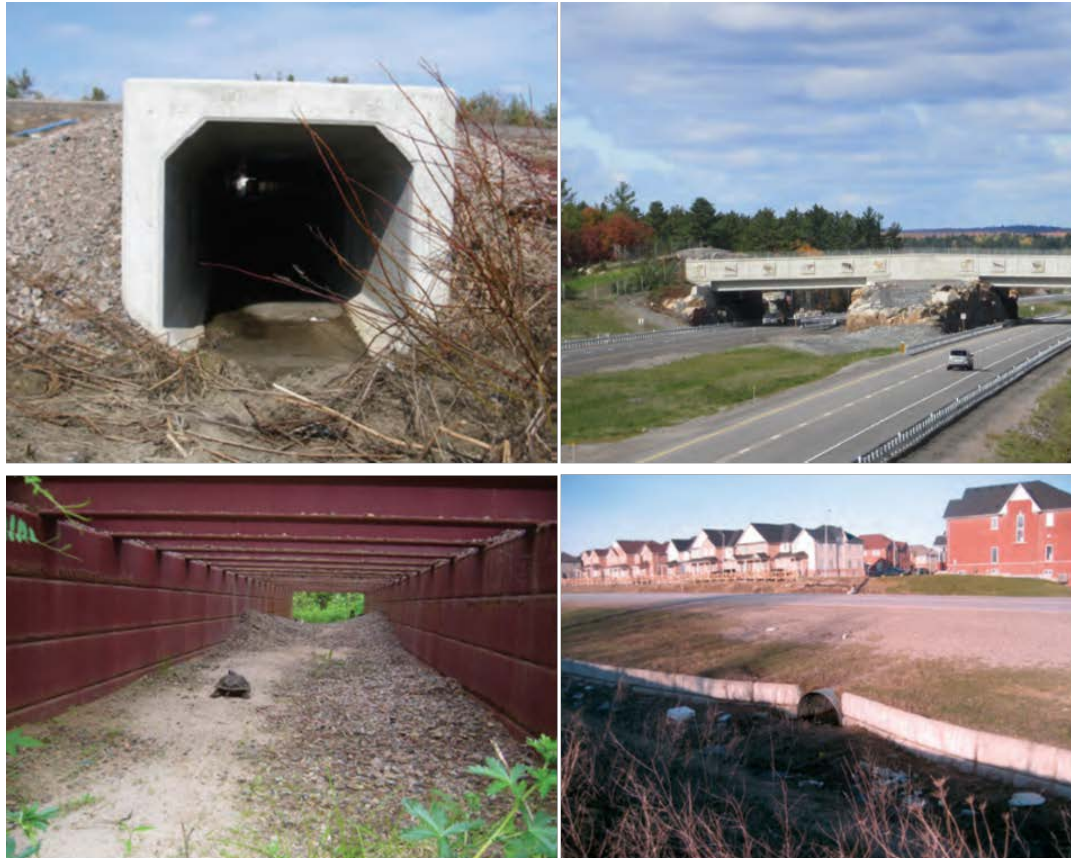
Figure 9: Images of examples of wildlife crossing structures in Ontario (top-left to bottom-right): box culvert underpass (©K. Gunson), 30m overpass on Hwy. 69 (©K. Gunson), open-grate tunnel (©A. Mui), concrete exclusion wall and culvert (©K. Gunson) (source: OREG, 2010)
