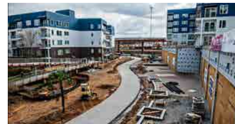
Figure 4.3.1.8 New construction on the Atlanta Beltline Trail paired with adjacent land development providing destinations for trail users Jonathan Phillips (2018)
