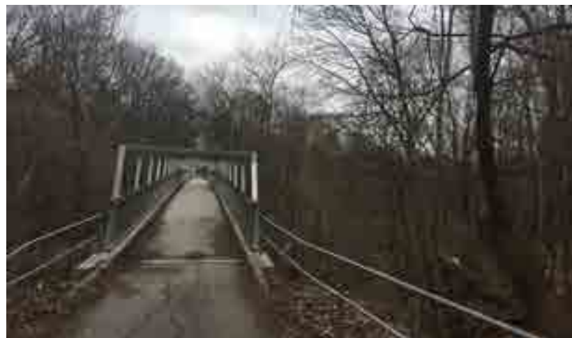
Figure 4.3.3.6 Pedestrian connection bridge across Mud Creek Toronto - April 10, 2019
