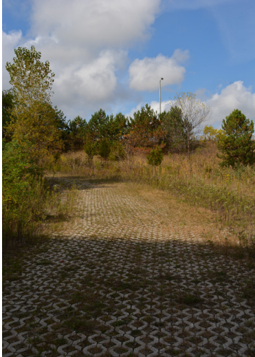
Porous paving stones found under the 401 overpass (Photo Source: Ketchabaw, 2013)
