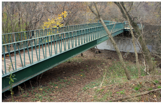
Pedestrian bridge extends beyond the banks of the river allowing wildlife to pass through
