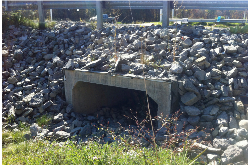
Box culvert for turtles, Ottawa, Ontario (Photo Source: Kluge, 2013)
