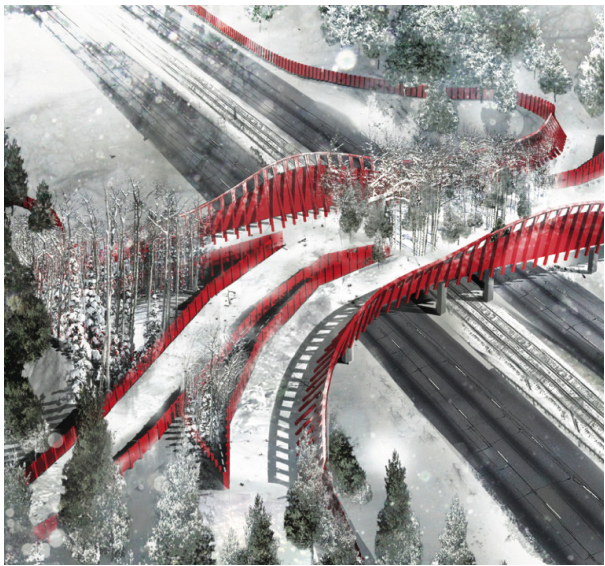
Figure 9 - Using red to highlight crossing structures can attract visual attention from road users, while not disturbing wildlife using the structures. (Image Credit: Janet Rosenberg & Studio Inc.)
