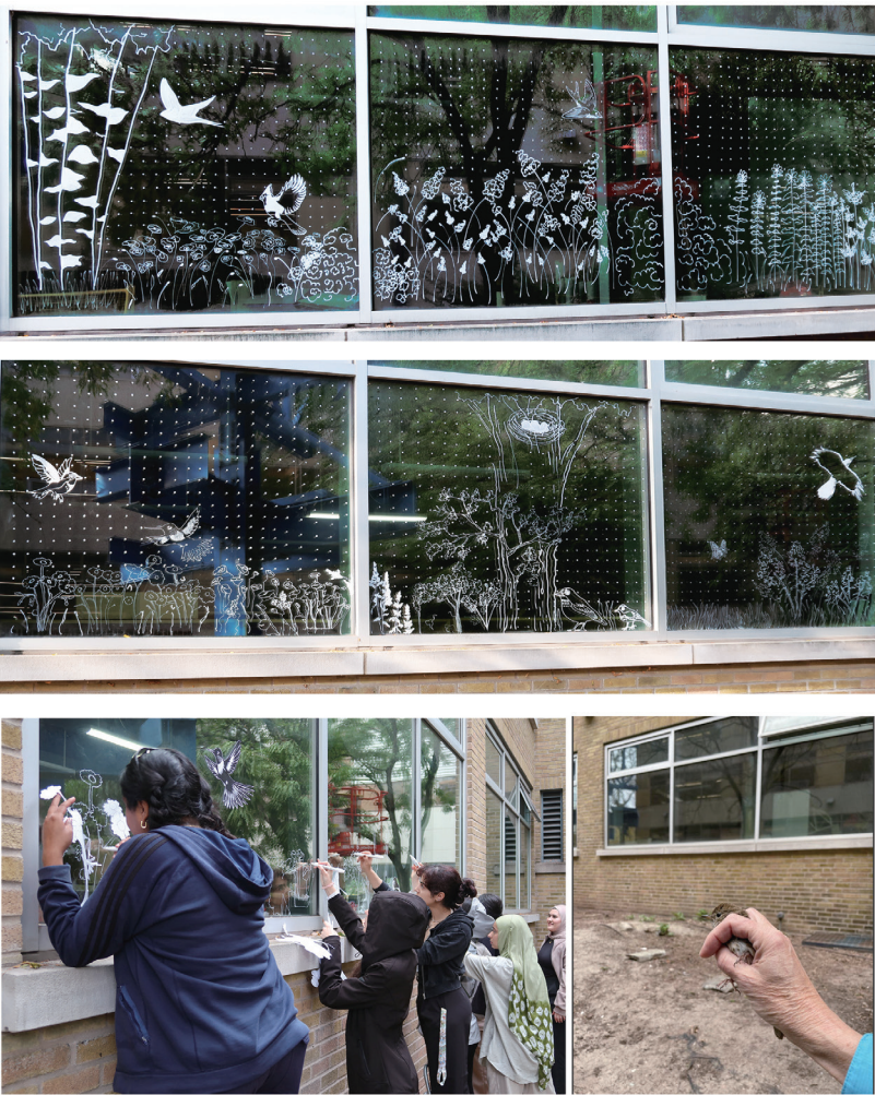
图 3 高碰撞风险建筑的鸟类友好临时窗面处理 Fig.3 Bird-friendly temporary window treatments at a collision-prone building
